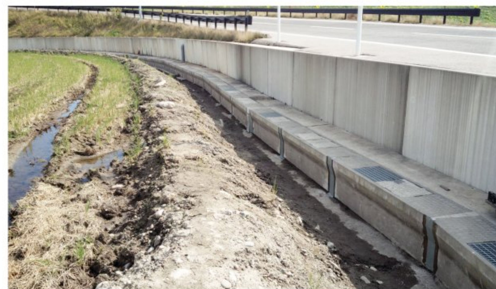
V S 側溝目地補修
